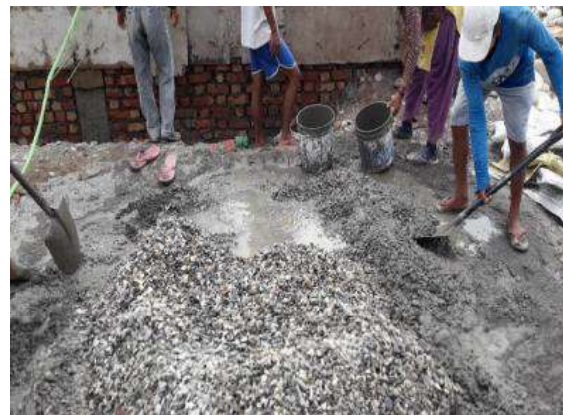
Figure 15. High water content for easy workability
