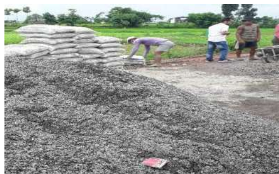
Figure 12. Impurities on Aggregate
