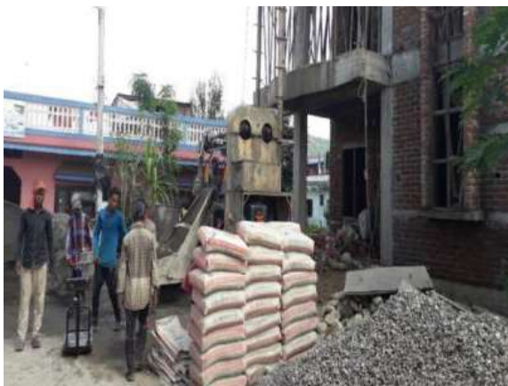
Figure 10. Stacking of Cement
