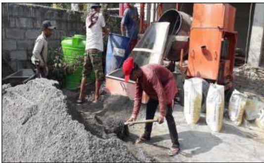
Figure 13. Worker feeding sand using shovel only
