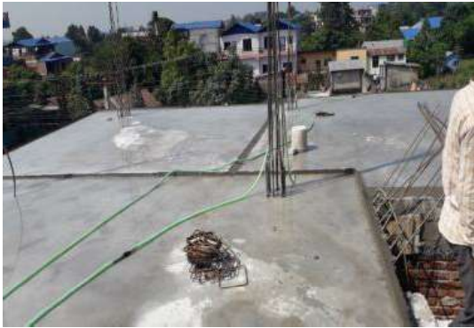
Figure 17. Work starting after 3 rd day of concreting
