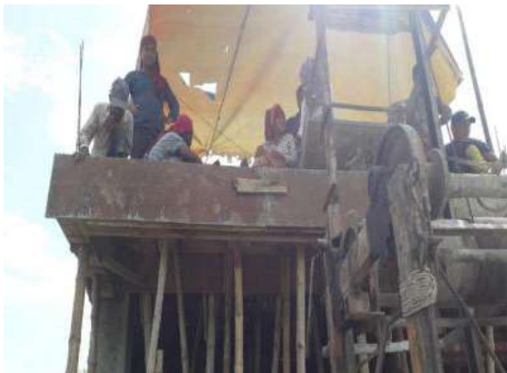
Figure 19. Use of Wooden props and wooden formwork
