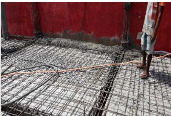
Figure 14. Concrete pouring segment wise in beam and slab portion
