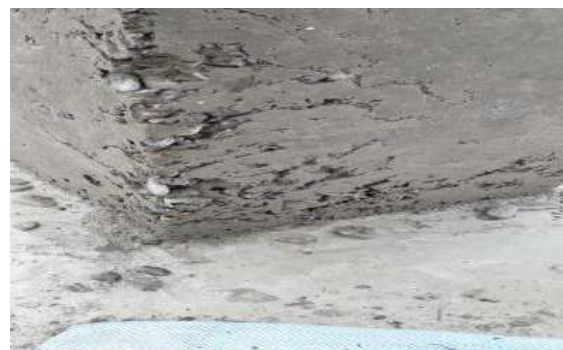
Figure 16. Improper compaction during concreting
